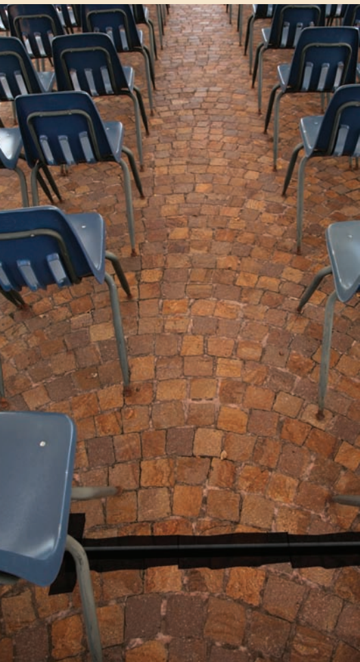
Figure 3 Use gaffer's tape for cables in traffic areas.
